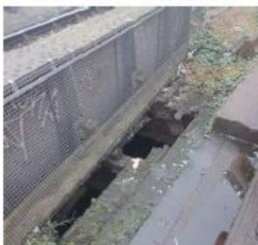
Decking Failure to West London Line Extension (BML1 2/14)
