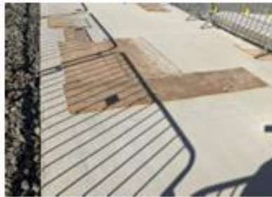
Photo showing the plywood boards covering the cable voids within the base
