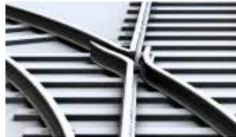
The Switch is the sliding part of the points, that determines which line the railway wheels are guided towards
