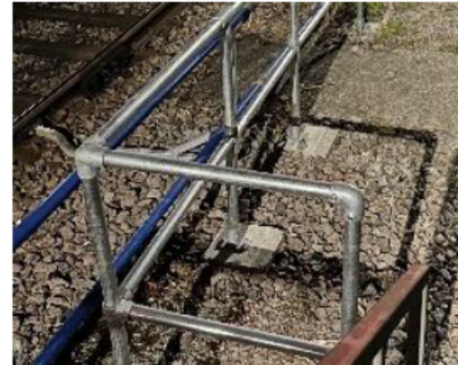
Vortok Fencing Installed behind the Permanent Handrail
