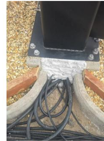
Fig 2: Pre-formed foam moulds held in place with fresh foam, behind which clay balls are installed in one visit
