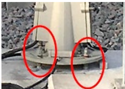
Figure 5 – Adjustment Studs
