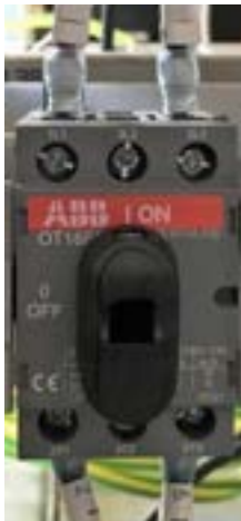
Figure 2 - ABB Power Switch OT16F3
