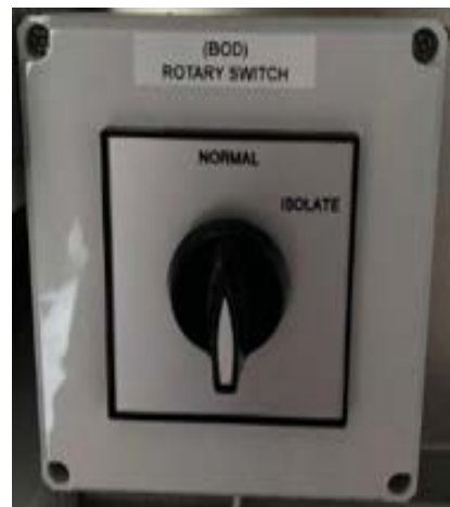
Figure 1 - Alstom BOD Rotary Switch
