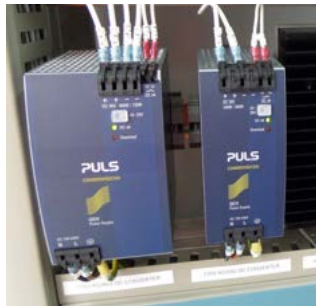
Figure 6 - AC-DC converters showing DC OK indication
