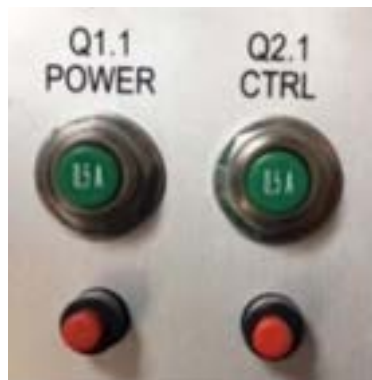
Figure 1 – Power and Ctrl Trips
