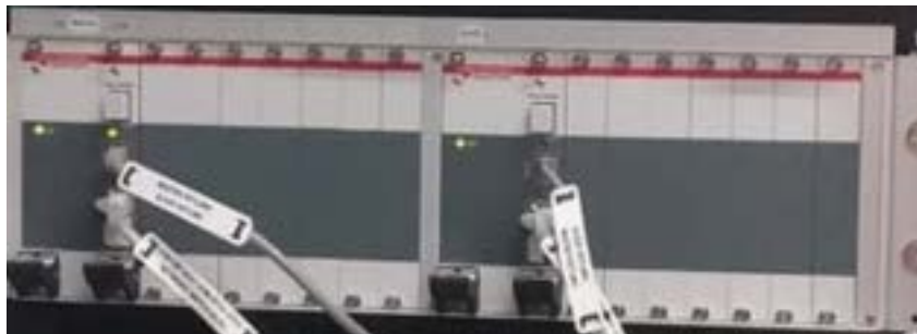
Figure 1 – Frauscher Concentrator 'Hotlink' Crossover Cable
