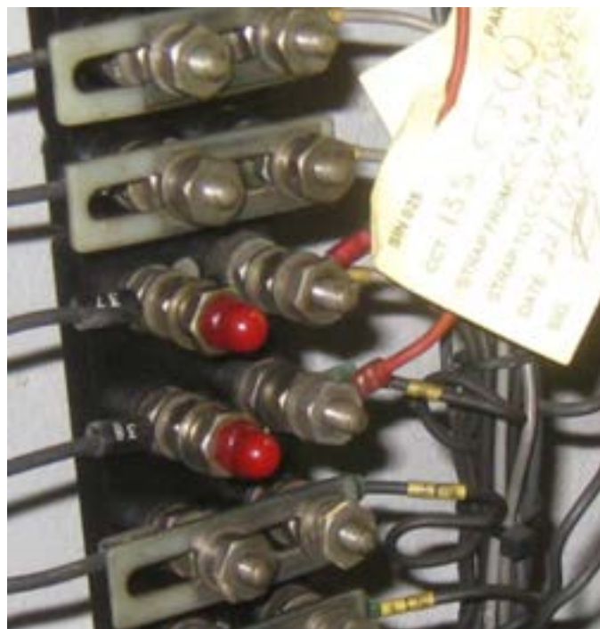
Figure 2 - Diversion Applied to a Terminal Block
