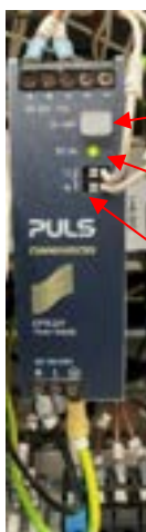
Figure 1 - CP10.241 Power Supply
