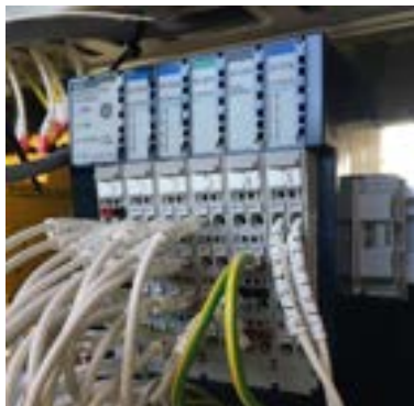
Figure 1 - Five RSTi ST Modules fitted to TCP-IP Network Adapter
