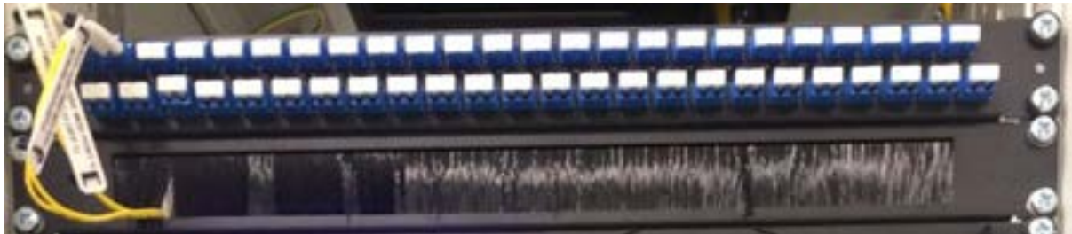
Figure 1 - Brandrex Patch Panel
