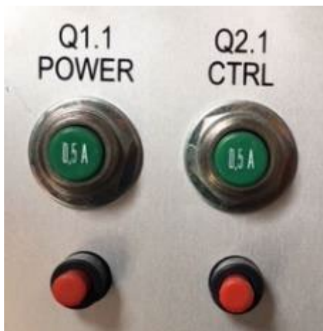
Figure 1 - Power and Ctrl Trips
