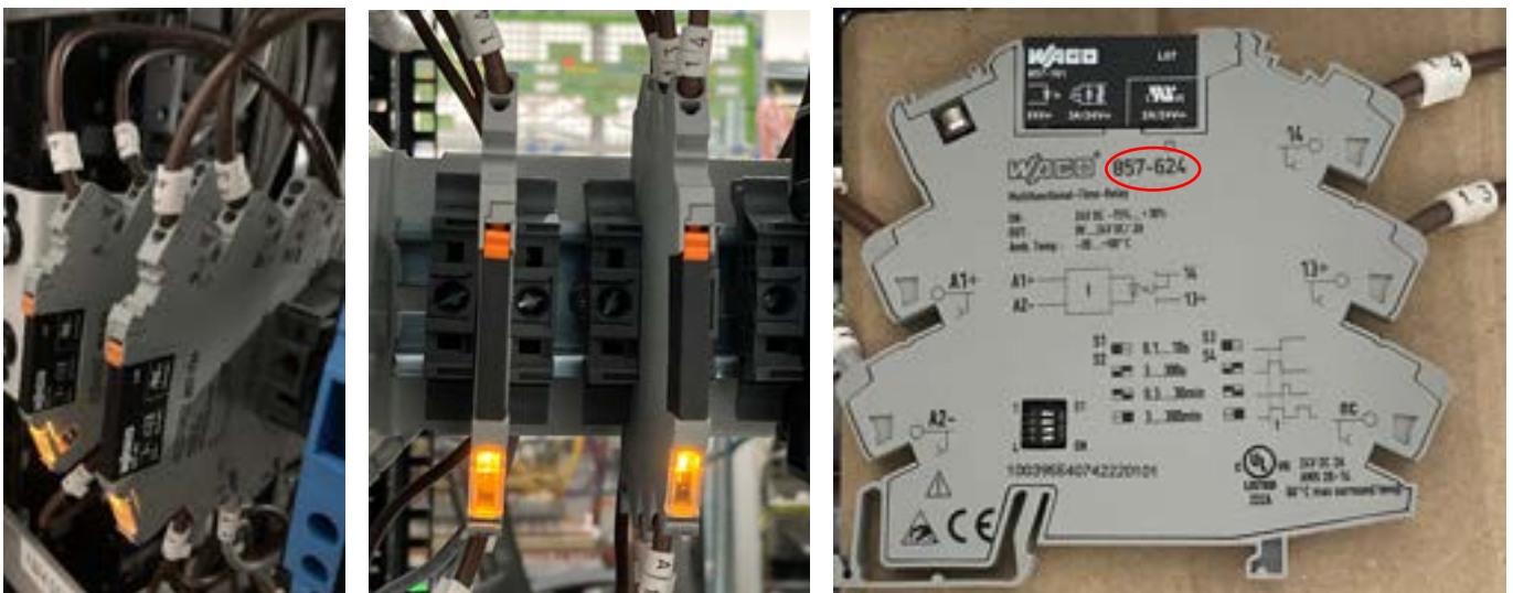
Figure 1 - A WAGO Multifunctional-Time-Relay 857 – 624
