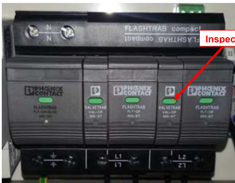
Figure 1 – FLASHTRAB mains surge protection
