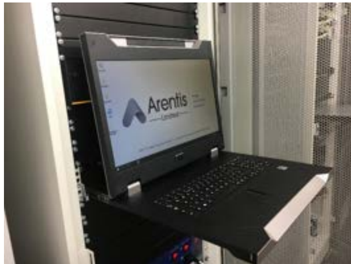
Figure 2 - KVM Monitor: Top view, extended position
