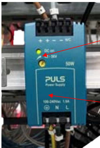
Figure 1 - ML50.105 Power Supply
