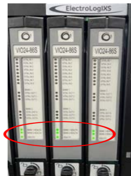
Figure 4 – I/O Health LEDs
