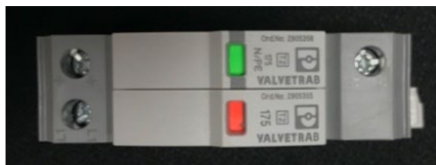
Figure 2 - Visual indication of an operational (green), and a blown Surge protector (red).
