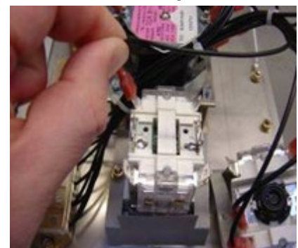
Figure 11 – Swapping Wiring to new contact block
