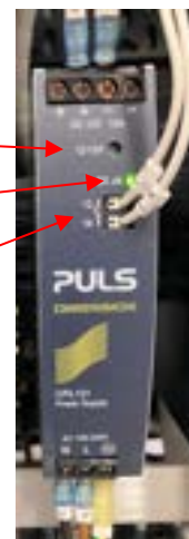
Figure 2 - CP5.121 Power Supply
