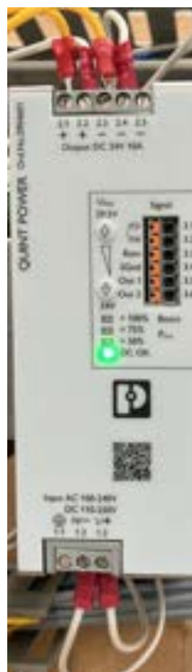
Figure 1 - QUINT-PS/24DC/24DC/5 Power Supply
