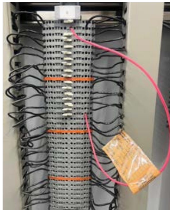
Figure 6 – Diversion Applied to a Wago using Method 2
