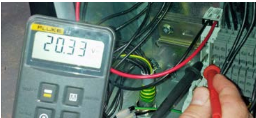
Figure 10 - Solar Panel Voltage measurement
