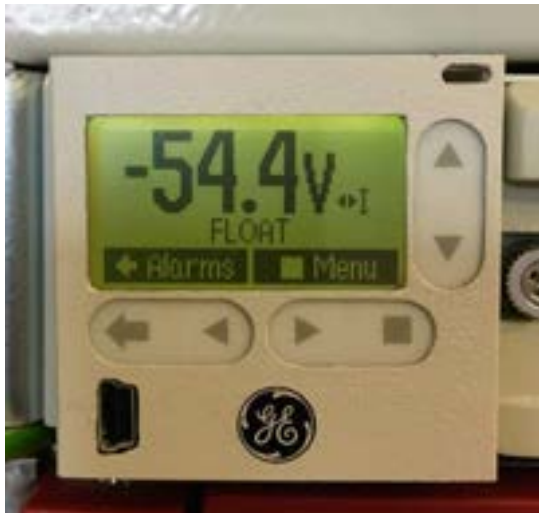
Figure 1 - Rectifier Controller Module (SPS841A_015R_D)
